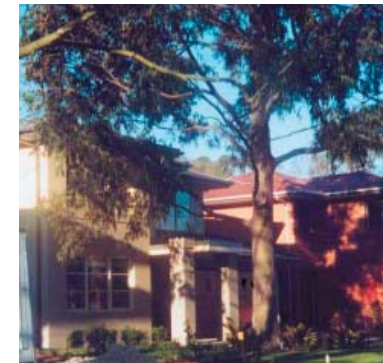
Combination of cladding & exposed brick
